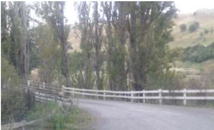
Figure 6.3b Bridge, Ruakokopatuna required structural assessment
